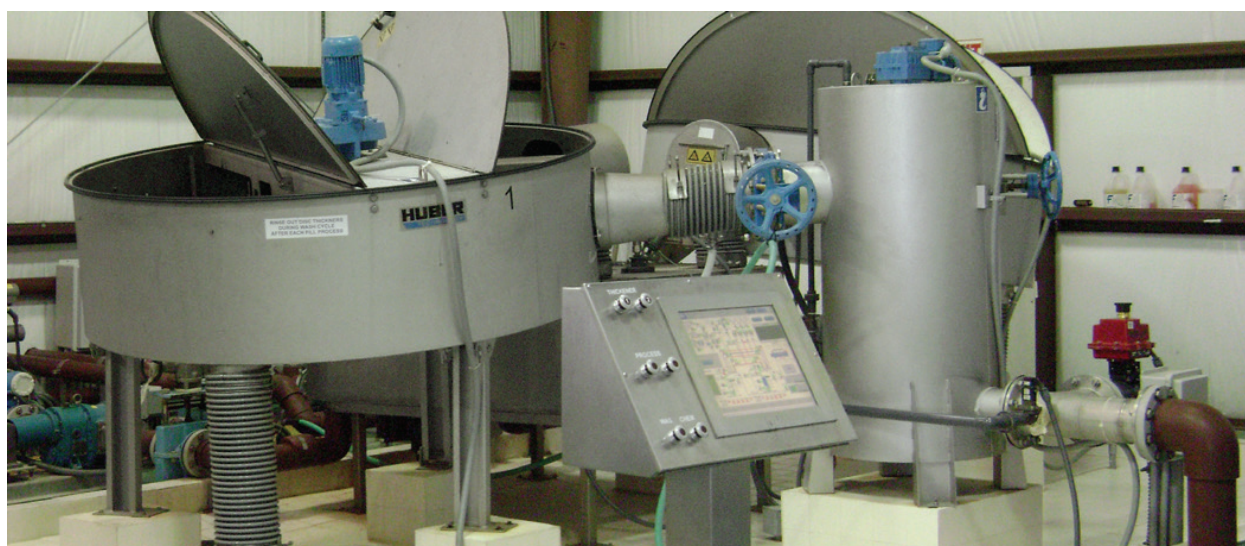
BCR's Neutralizer® solution incorporates Huber's easy-to-operate HMI and disk thickeners that simplify use and reduce energy consumption and costs.
